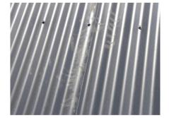
Figure 2. Roofing with sunscreen damage
